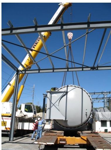
One of the new autoclaves being installed at North Coogee
